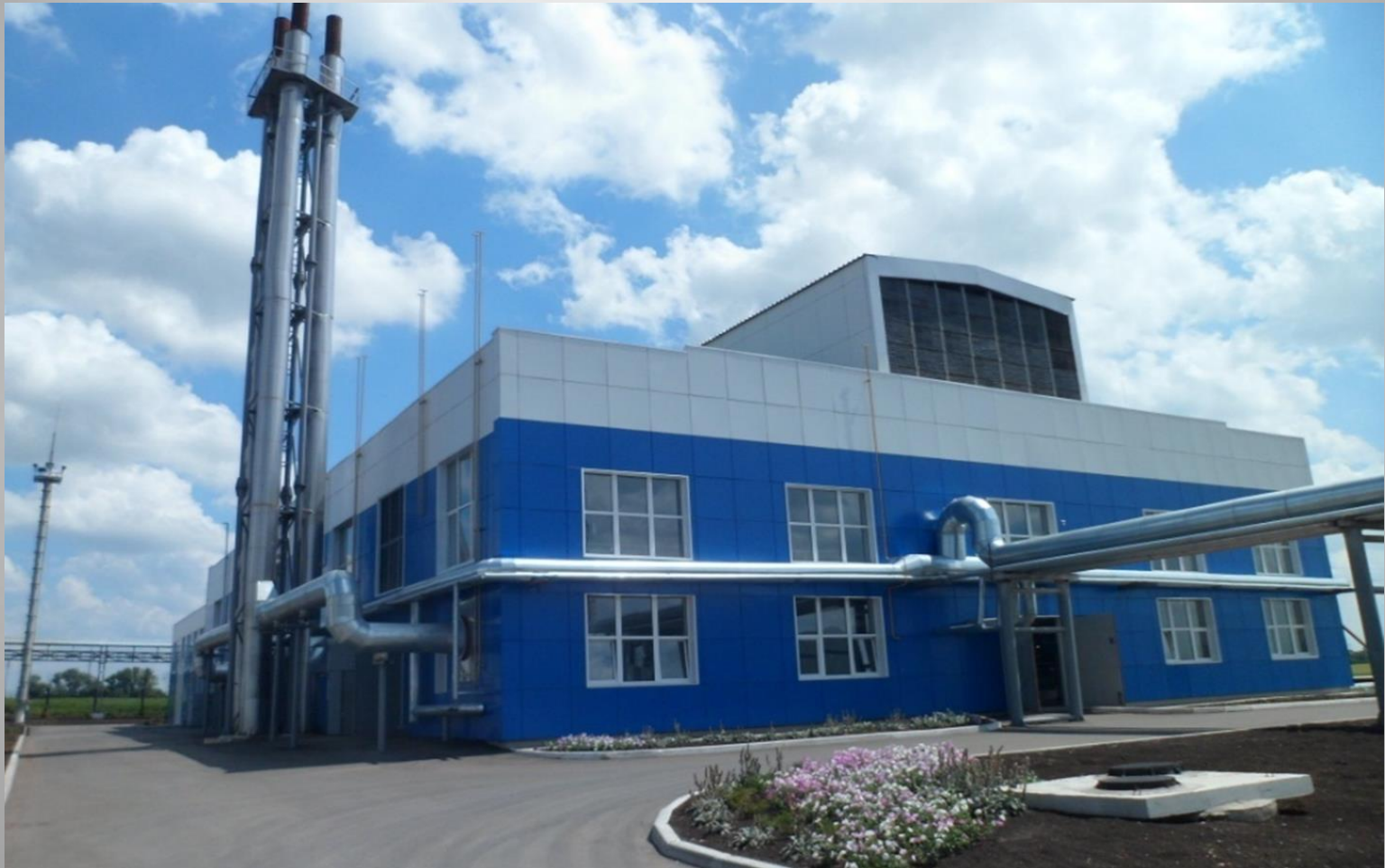
Coalmine “Pokrovskaya”, 75 MW el
