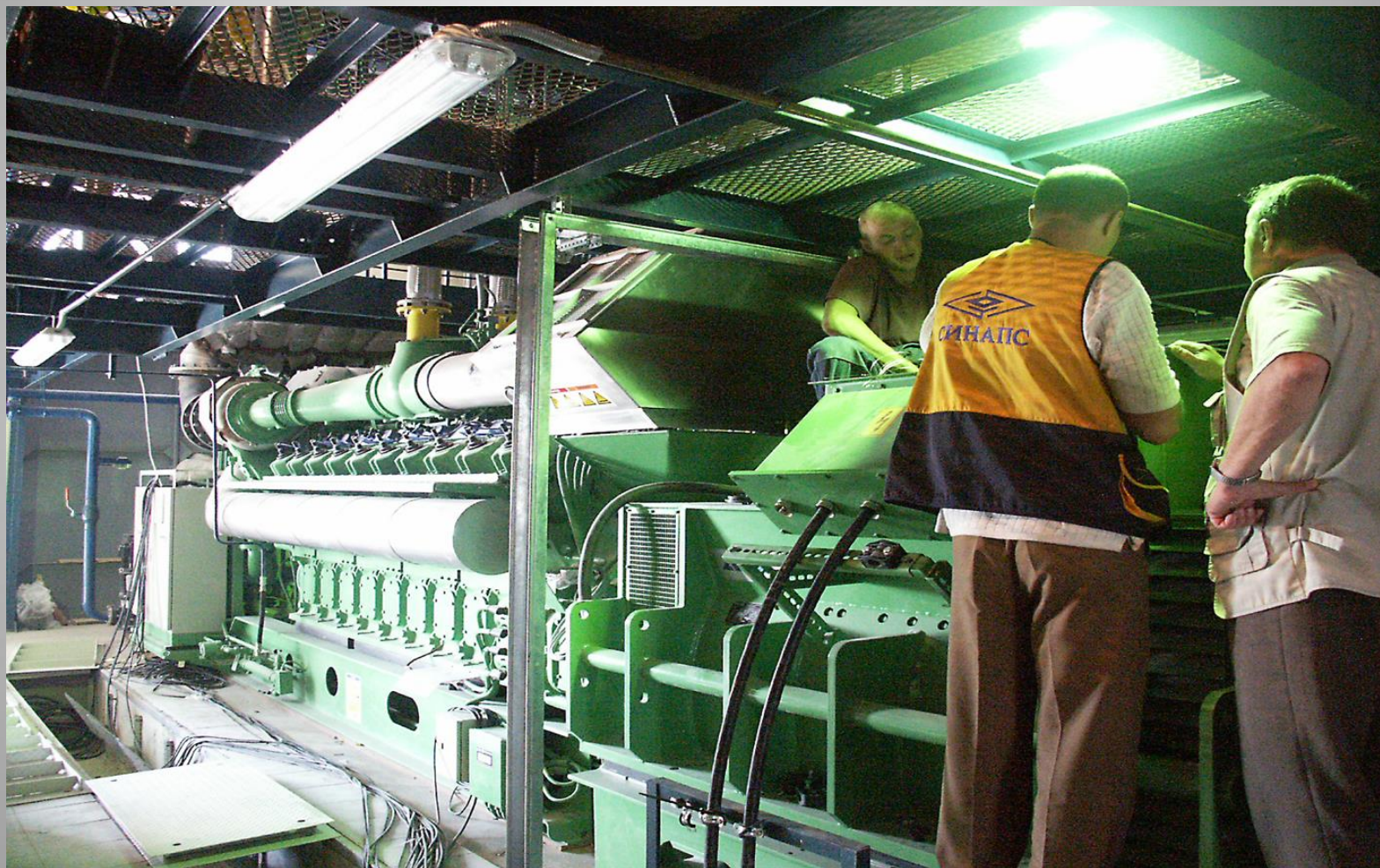
Coalmine "Pokrovskaya", 75 MW el
